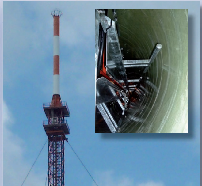
VHF DAB+ transmitting antenna in "Saarbrücken" GRP cylinder
