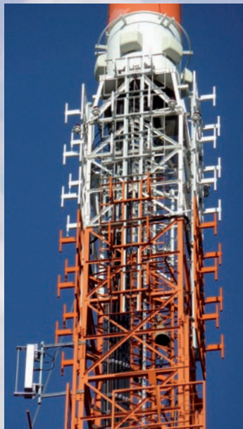
VHF DAB+ "Heidelberg" transmitting antenna
